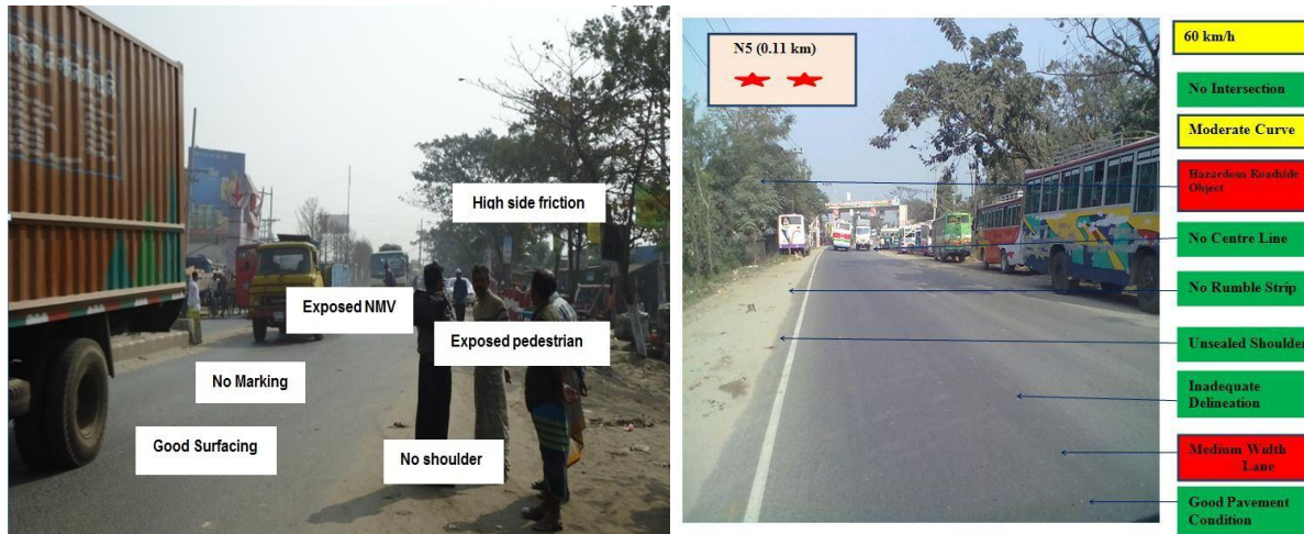
Figure 2: Typical sections of N5 Highway rated 2-stars.
