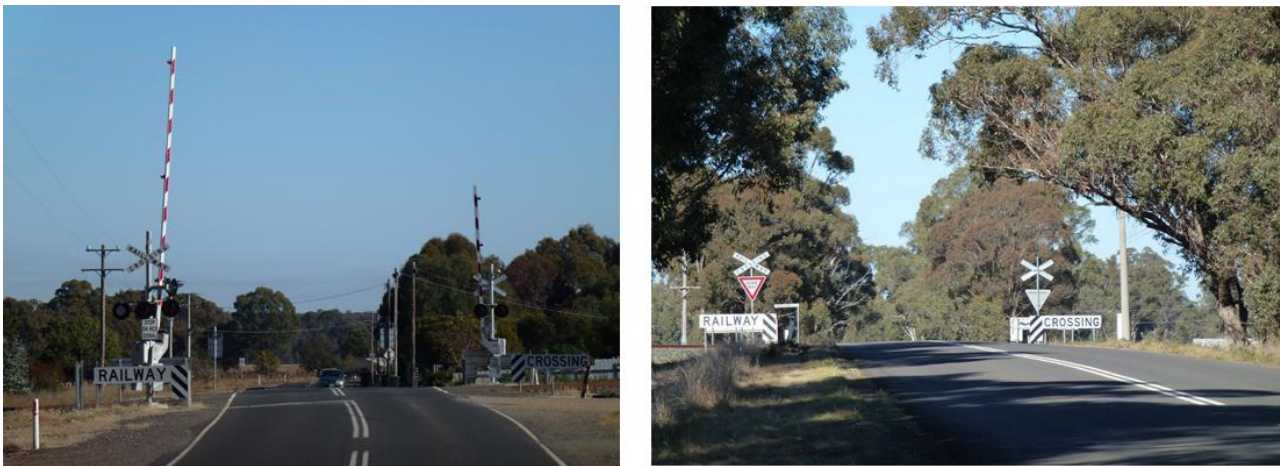
Figure 2. Images for an active (left) and passive (right) RLX in the study route
