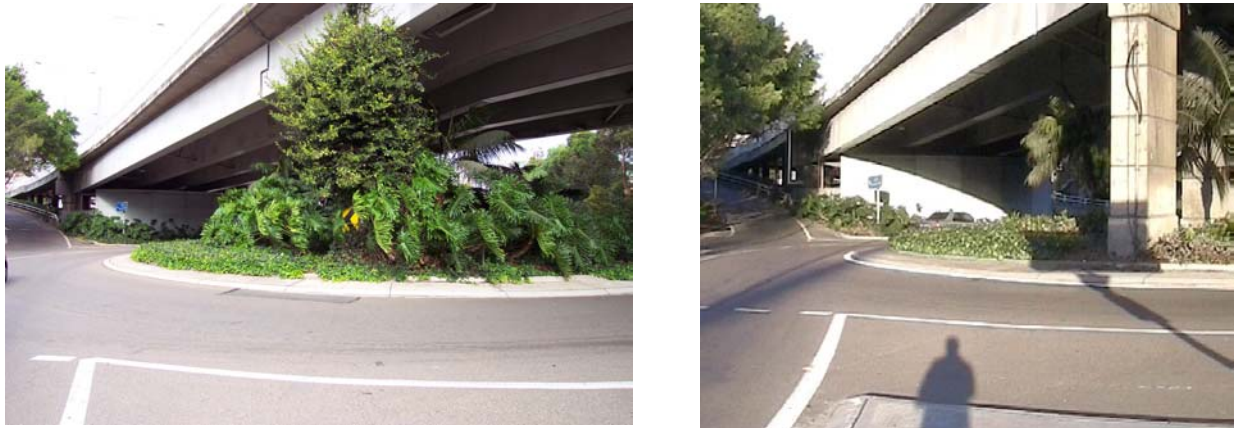
Figure 10a (left) and 10b (right): The sight-obstructing vegetation shown in the photo on the left was removed to improve sight distance through the intersection. Work completed on 10 June 2003.
