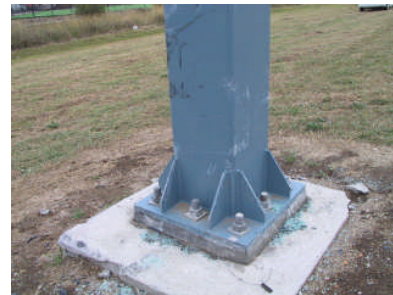
(i) Case 4: Base of the road sign pole.
