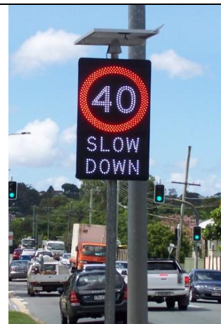
Vehicle activated "SLOW DOWN" speed limit sign (installed in conjunction with static school zone sign)
