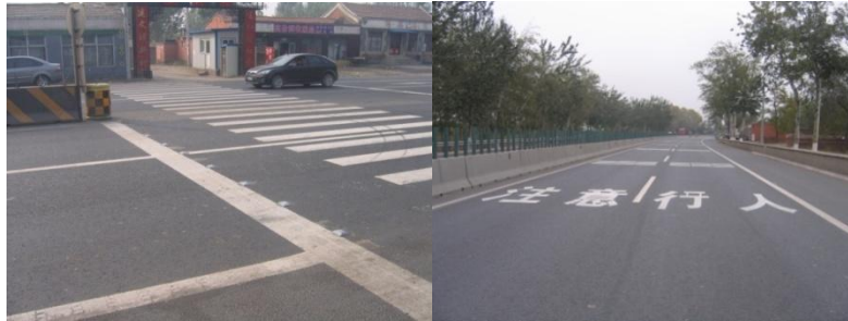
Figure 16 pedestrian crossings with colored anti-skid pavement
