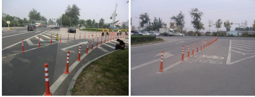
Figure 13 channelization on pavement modified with poles Figure 14 poles to separate non-motor vehicles from motor vehicles
