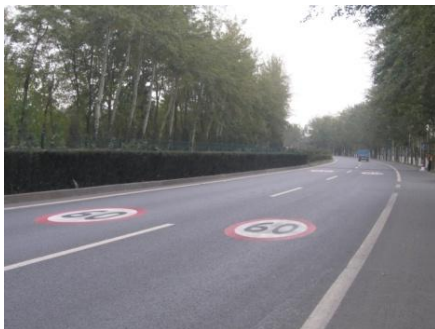
Figure 11 “Gate” at the beginning of the speed zone
