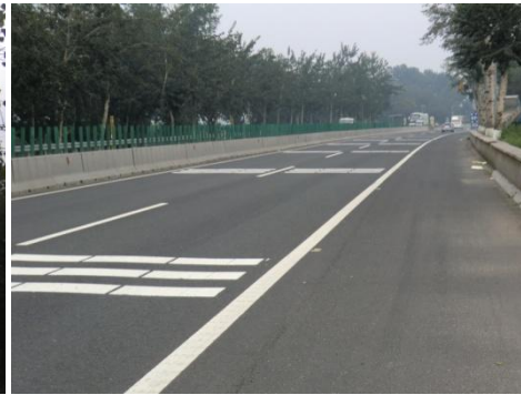
Figure 8 Horizontal Pavement Marking
