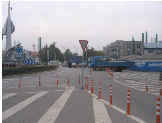
Figure 15 “YIELD” and “STOP” signs and markings installed
