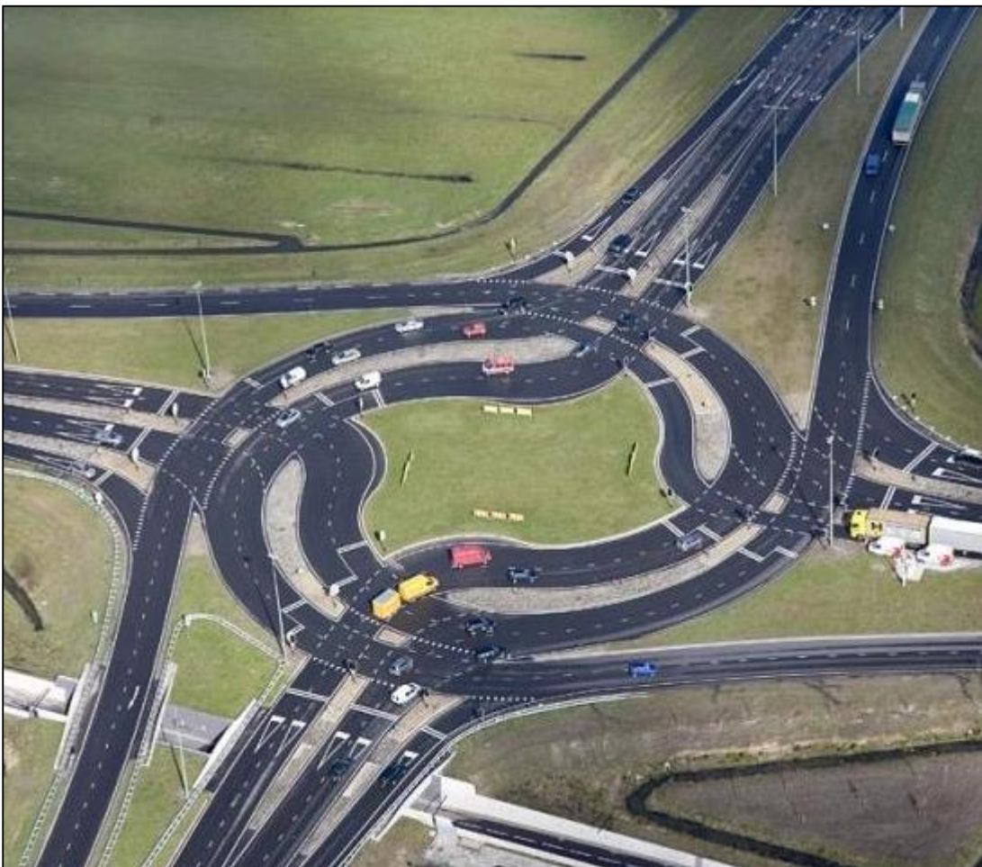
Figure 3 – Turbo-roundabout north of Rotterdam in the Netherlands
