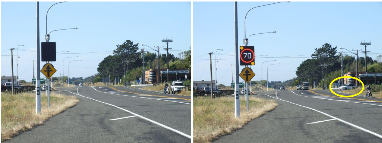
Figure 1. The RIAWS in operation at Himatangi with no conflict risk (left) and a potential conflict risk (right) with a side road vehicle present (circled).
