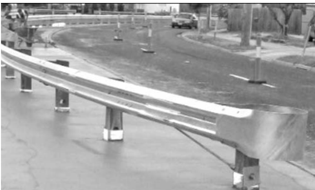
Figure 15: Example of typical W-beam guardrail (manufactured by Armco)
