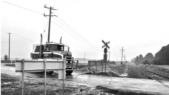
Figure 3: View of the Trawalla level crossing showing a prime mover stopped at the crossing (part of the DVE incident investigation and reconstruction). Note the acute angle of the crossing to the roadway.
