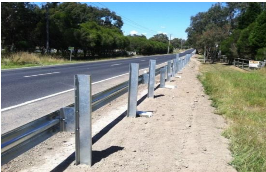
Figure 3. Posts not embedded to the correct depth from Cassar (2015)
