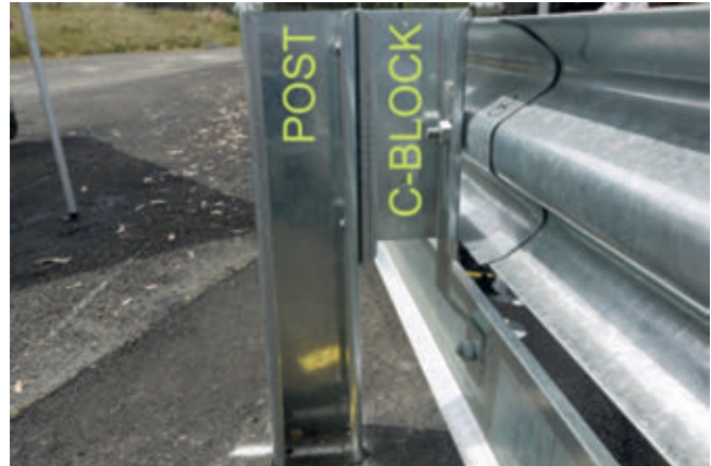
Figure 6. The public domain MPS attached to the W-Beam barrier
