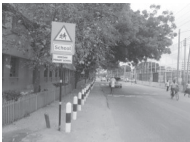
Figure 5. Low cost infrastructure measures – Bollards and Signage
