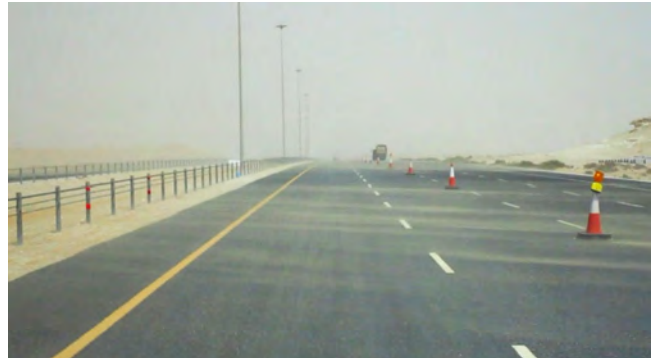
Figure 12. No sand accumulation with two-row wire rope barriers
