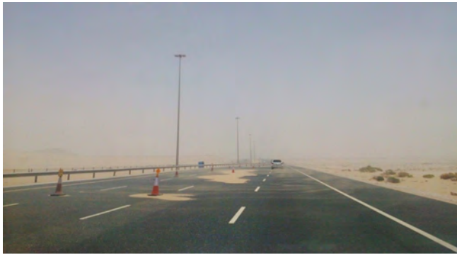
Figure 11. Sand accumulation with a split wire rope and steel W-beam barrier configuration
