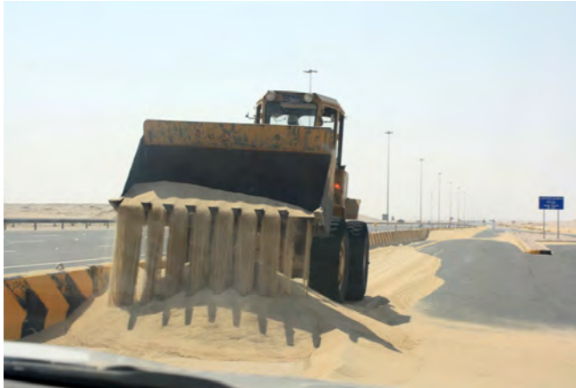
Figure 5. Example of sand accumulation associated with a concrete barrier
