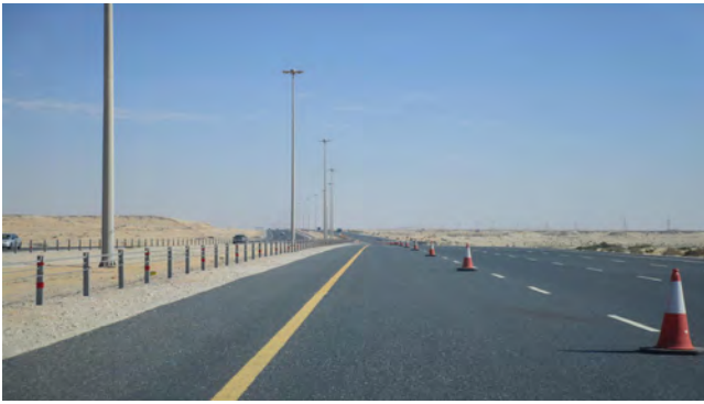
Figure 8. Wire rope barrier installation (August 2015)
