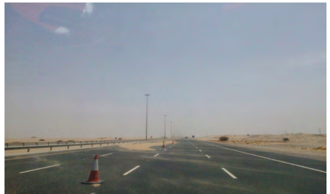
Figure 10. Sand accumulation with existing two-row steel W-beam barriers
