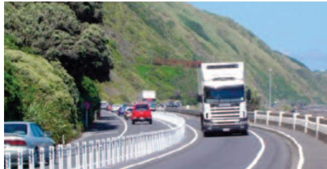
Figure 4. An example of the Coast Road median barrier in New Zealand (Photo courtesy of the New Zealand Transport Agency)
