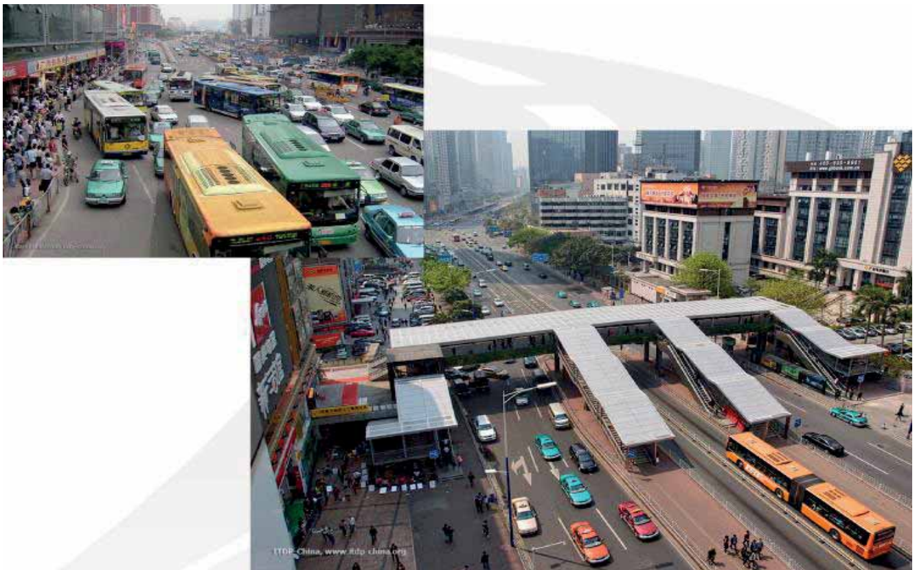
Figure 1: The contrast of congestion and risk created by curbside bus operations versus a well-designed BRT system
