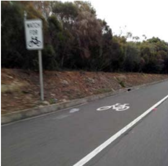
Figure 1. Typical motorway sealed shoulder treatment
