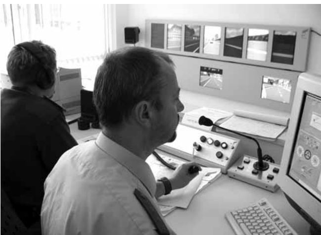
Fig. 3: Control Room with Monitors for Co-driver and Instructor
