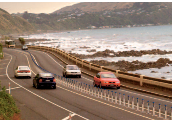
Figure 5. Narrow median wire rope barrier installation on Centennial Highway
