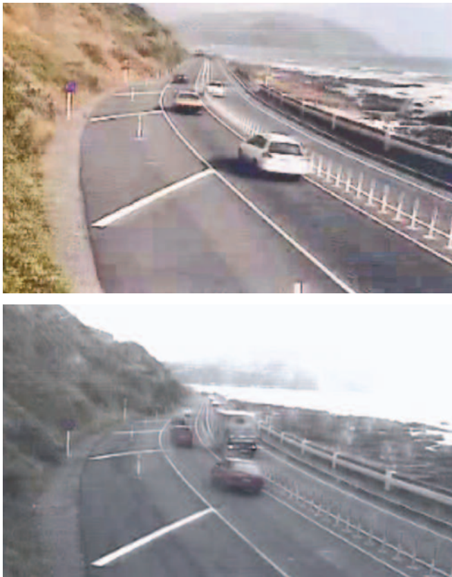
Figure 7. Two separate incidents involving vehicles hitting the median barrier
