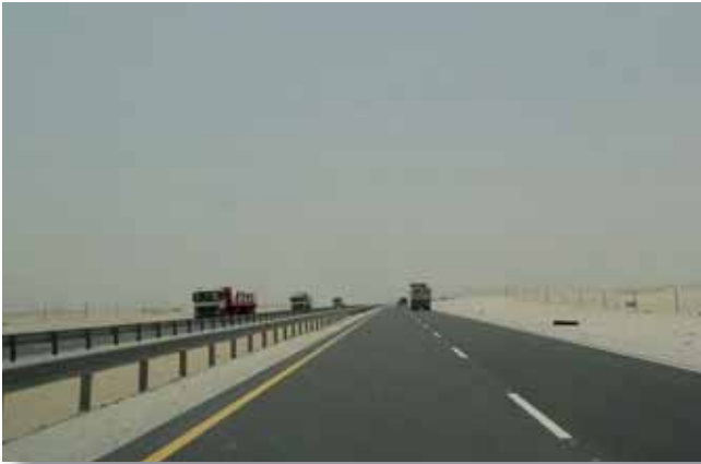
Figure 5. Route 55 after the upgrade
