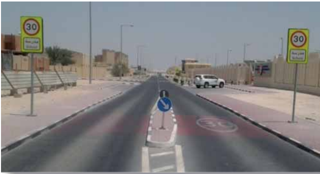
Figure 2. School zone gateway treatment at London School
