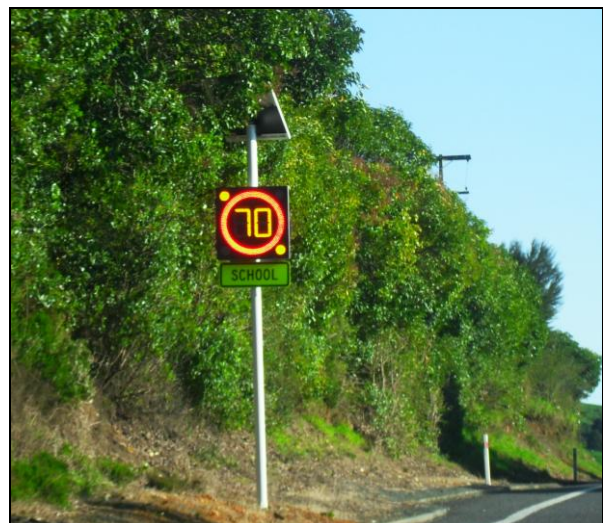
Figure 6: 70km/h variable speed limit school trial sign on State Highway 27 at Kaihere School (within permanent 100km/h speed limit).
