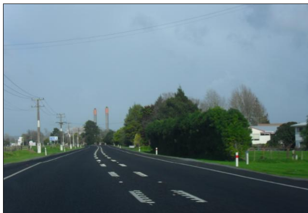
Figure 1: Wide centreline markings on State Highway 1 north of Huntly where passing is permitted
