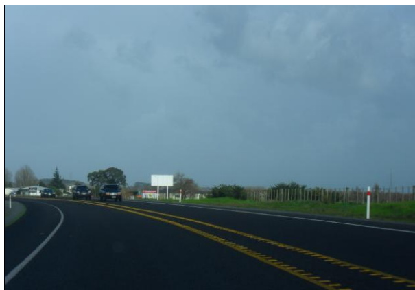
Figure 2: Wide centreline markings on State Highway 1 north of Huntly where passing is not permitted
