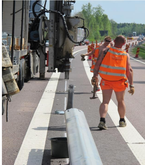
Figure 3. Specialised barrier installation equipment.
