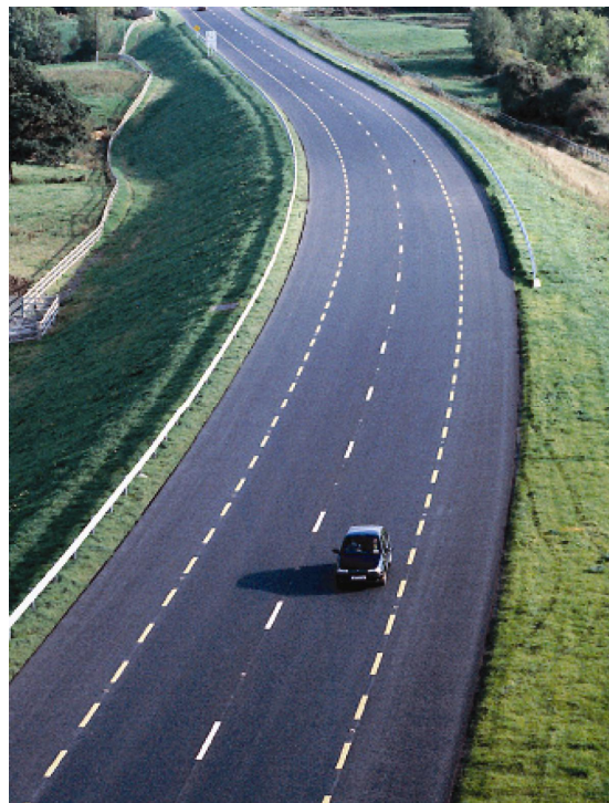
Figure 1 Wide single carriageway design in Ireland
