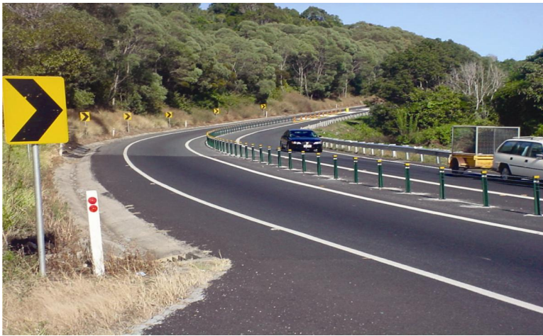
NSW Pacific Highway: St Helena
