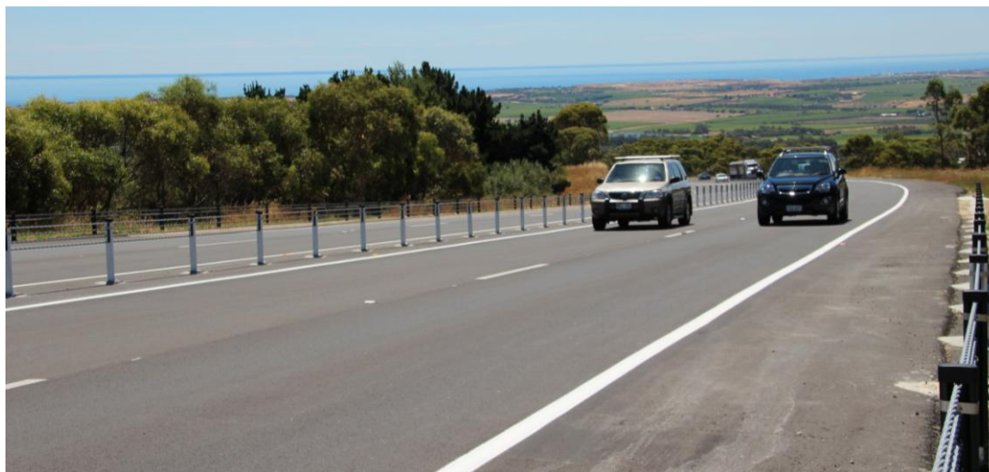
Figure 3 View of median wire rope barrier at Willunga Hill, looking north
