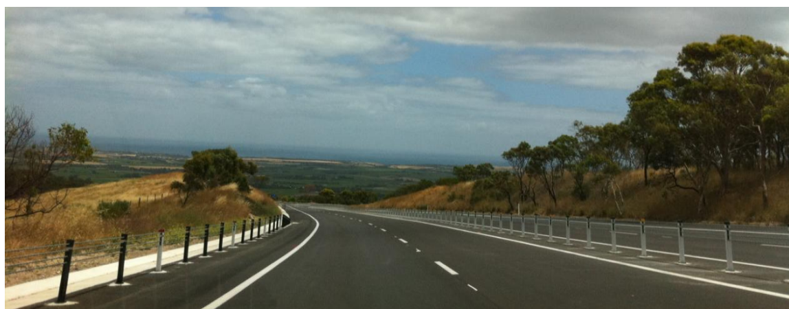
Figure 4 Median and roadside wire rope barrier at Willunga Hill, looking north
