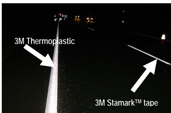
Figures 6-7 3M™ All Weather Thermoplastic and Stamark™ tape application on Mona Vale Rd, St Ives, NSW
