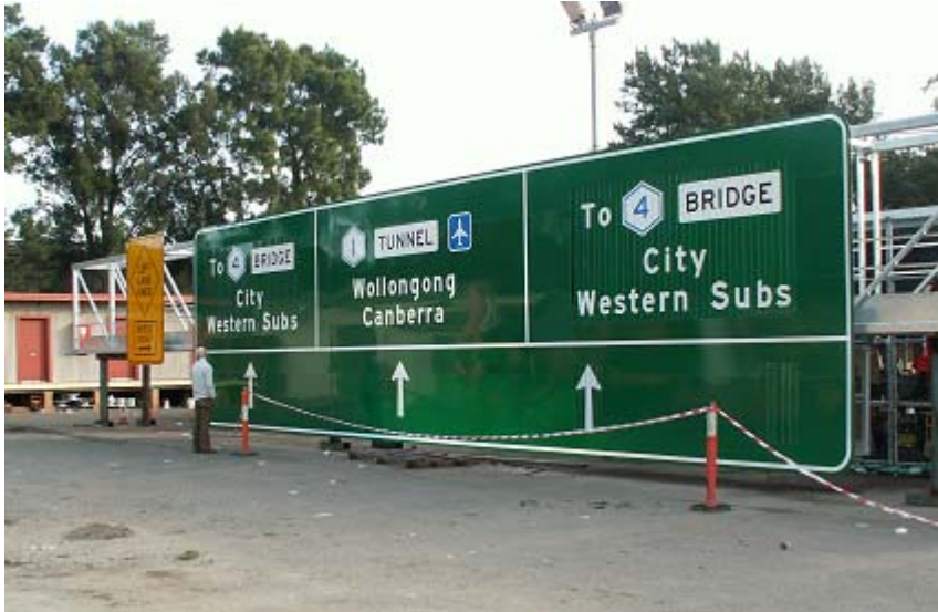
Figure 3 – Class 1X guide sign with 3M™ Diamond Grade™ DG3 sheeting
