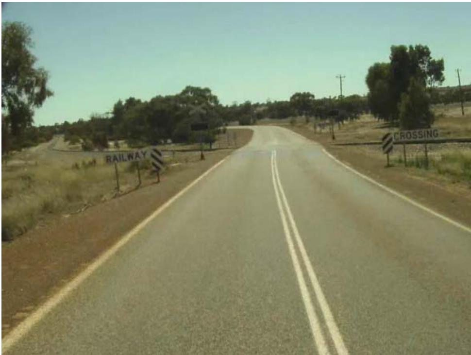
Figure 2 Railway level crossings on Goomalling Merredin Road
