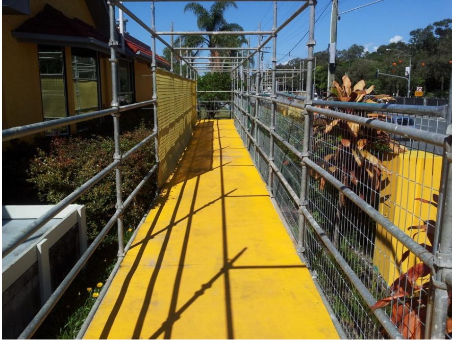
Figure 6 - Temporary Pedestrian Structure
