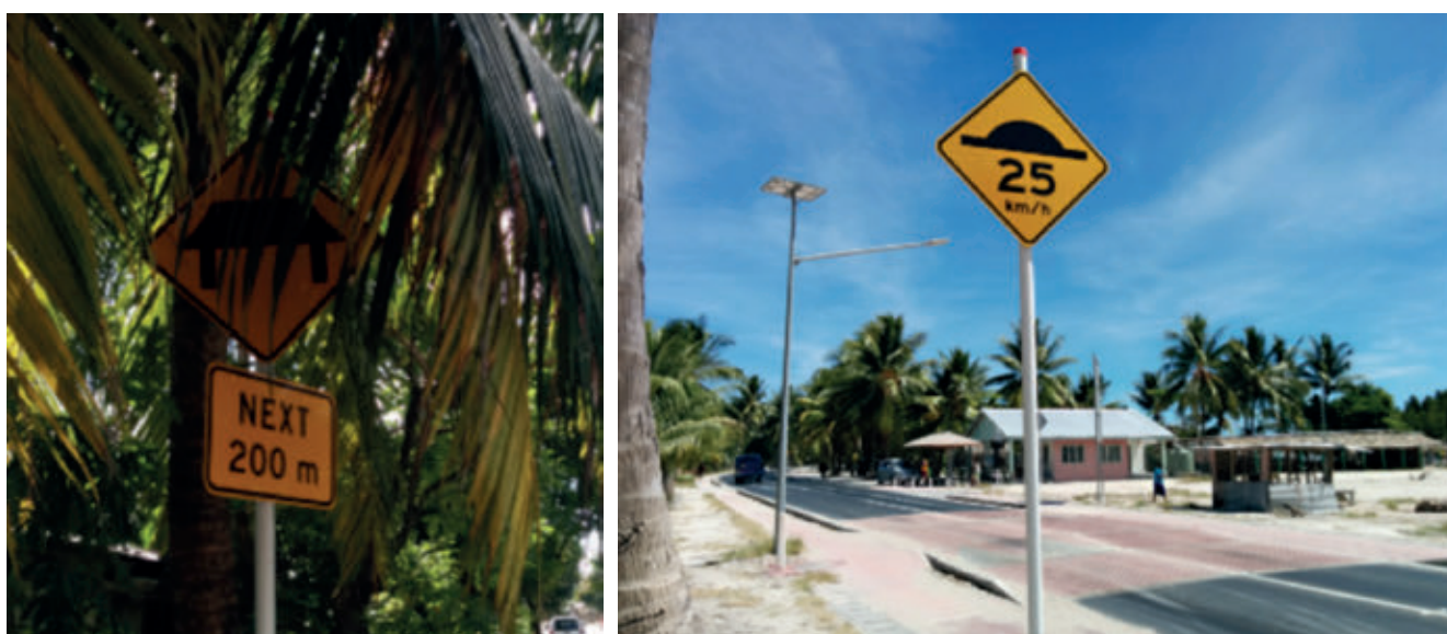
Figure 7. Example of obscured signage (left) and completed road showing safety features including signage, line marking, lighting, speed humps, footpaths and drainage (Whalley, 2017)
